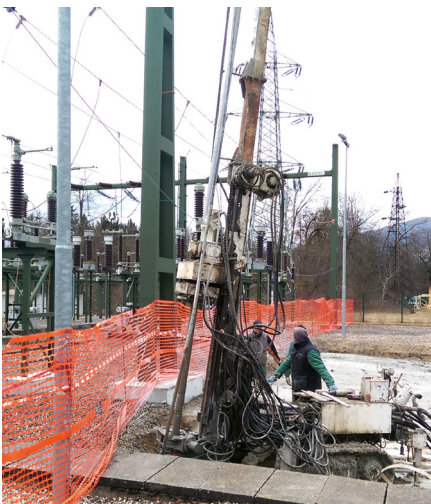
Vgradnja jet grouting pilotov
